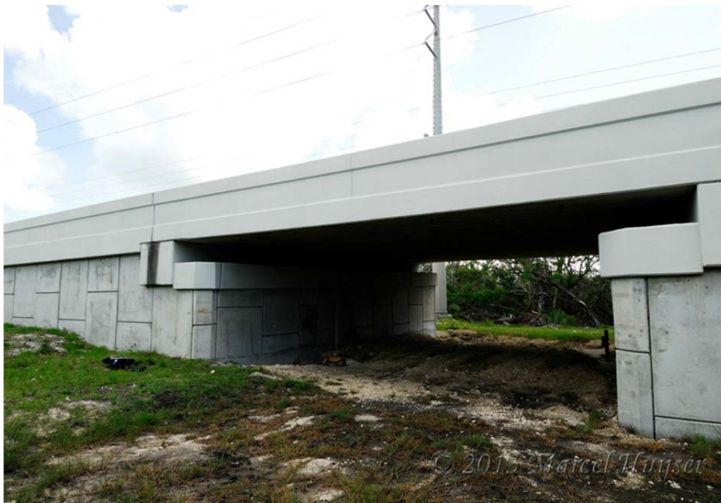
Figure 27: An underpass (14 m wide, 3 m high) designed for Florida Key deer ( Odocoileus virginianus clavium ) along US Hwy 1, Big Pine Key, Florida, USA (© Marcel Huijser).
