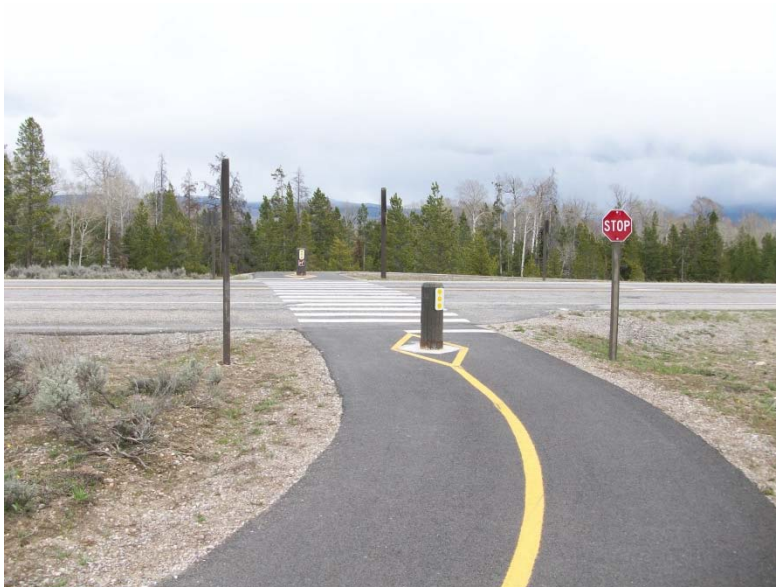
Figure 32: Example of bollard and sign post to prevent auto use of bike path (Source: Pat McGowen).
