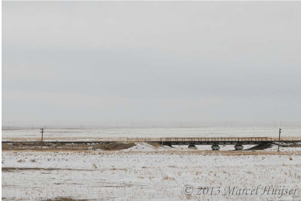
Figure 9: Underpasses for livestock and/or water along Trans-Mongolian Railway, between Choyr and Nalayh, Töv / Govisumber, Mongolia (© Marcel Huijser). The railroad and the livestock fence are a substantial barrier to the movements of khulan and Mongolian gazelle. The underpasses, bridges and culverts are not or barely used by these species as they are likely to small (not wide enough, not high enough).
