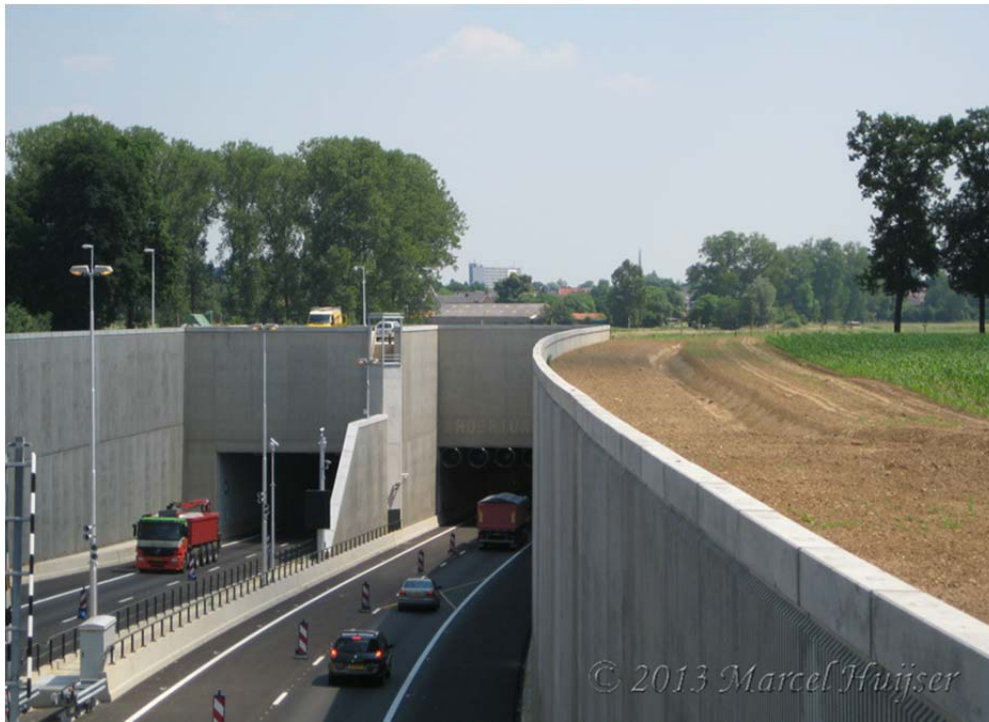
Figure 21: Landscape bridge Roertunnel, A73 motorway near Roermond is tunneled for 2.5 km under a small scale agricultural landscape and small river (Roer) and an urban area, near Roermond, The Netherlands (© Marcel Huijser).
