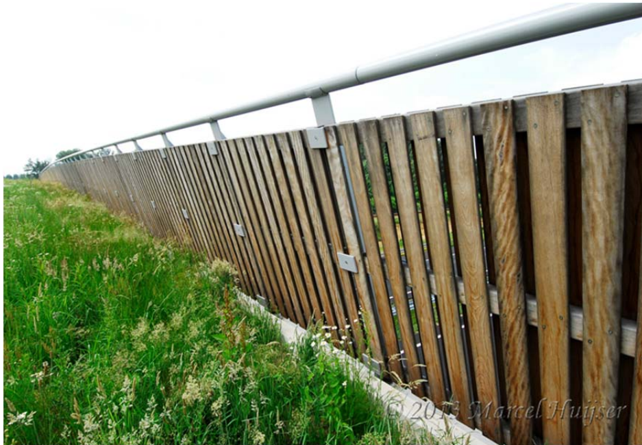
Figure 28: Wildlife fence and visual barrier integrated into one structure on top of wildlife overpass, The Netherlands (© Marcel Huijser).
