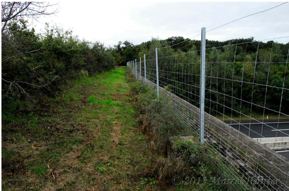
Figure 29: Wildlife fence (physical barrier) on the right and earthen berm with shrubs (visual and sound barrier) on the left on top of wildlife overpass, Austria (© Marcel Huijser).
