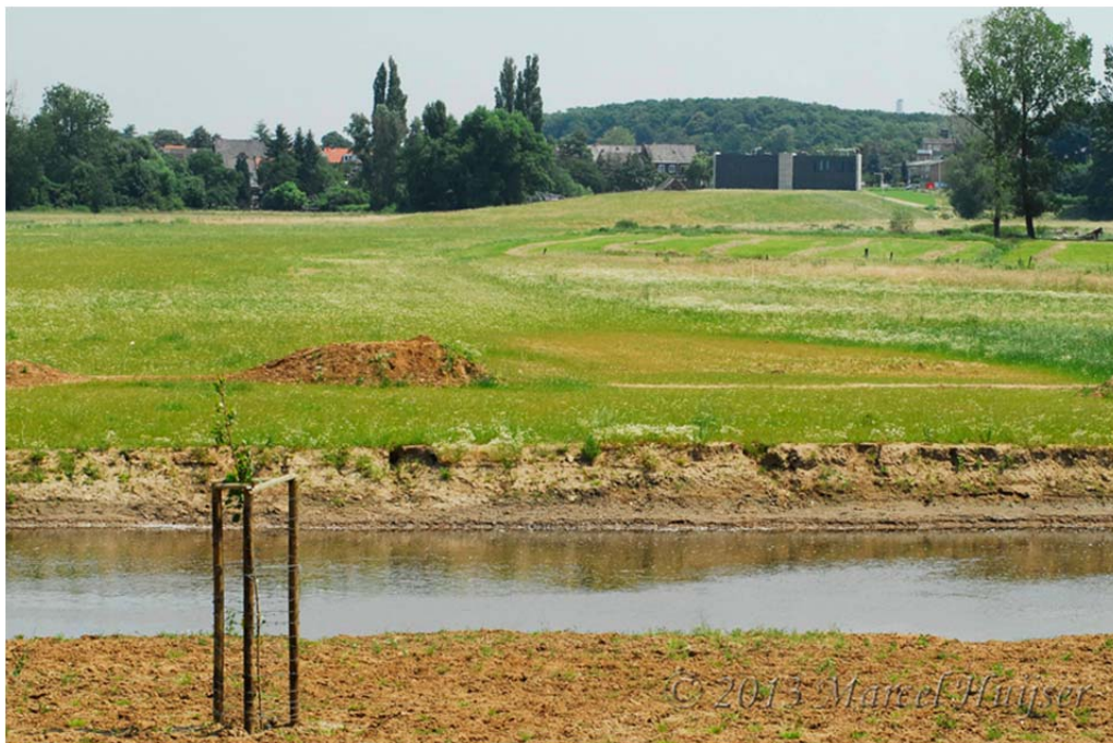
Figure 22: Another view of the Landscape bridge Roertunnel, A73 motorway near Roermond, The Netherlands (© Marcel Huijser). This image is taken on top of the landscape bridge. The dark rectangle in the background is part of the tunnel structure.
