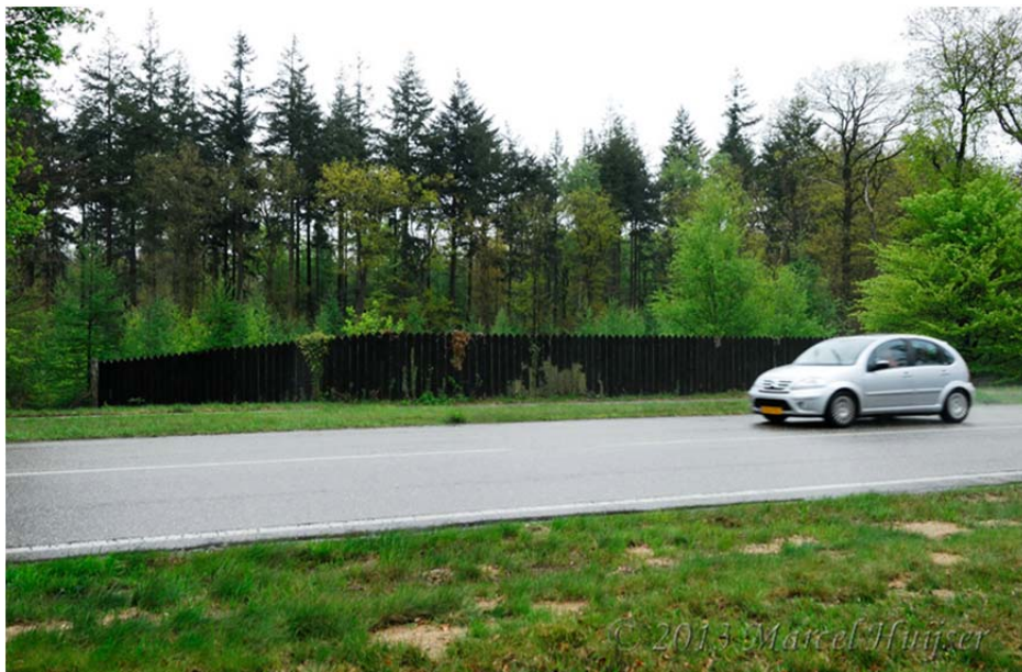
Figure 11: Visual barrier above wildlife underpass, near "Aardhuis" along N344, Amersfoortseweg, Hoog Soeren, The Netherlands (© Marcel Huijser). Note that the visual barrier along the project road in the Gobi should extend hundreds of meters beyond the actual crossing structure because of the open landscape, long view distances, and the road avoidance behavior of the desert ungulates.
