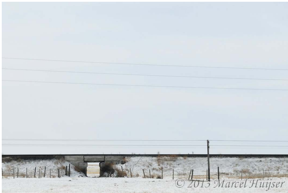
Figure 8: Underpasses for livestock and/or water along Trans-Mongolian Railway, between Choyr and Nalayh, Töv / Govisumber, Mongolia (© Marcel Huijser). The railroad and the livestock fence are a very substantial barrier to the movements of khulan and Mongolian gazelle. The underpasses, bridges and culverts are not or barely used by these species as they are likely to small (not wide enough, not high enough).
