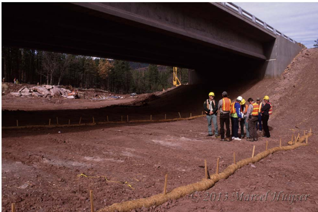
Figure 26: An underpass, likely several dozens of meters wide, designed for elk ( Cervus canadensis ) Tonto National Forest, Arizona, USA (© Marcel Huijser).
