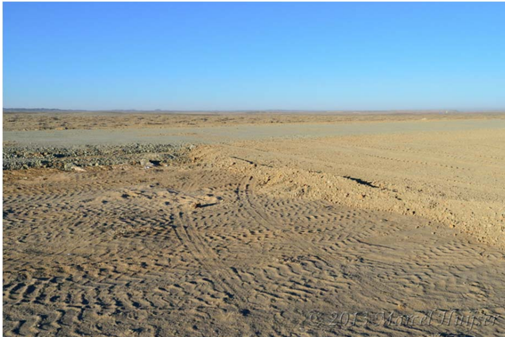
Figure 6: Livestock crossing along OT-GS Road, Gobi, Ömnögovi, Mongolia (© Marcel Huijser). A livestock crossing consists of a very gradual slope on both sides of the road (perhaps about 10-20 m wide (road length) at selected locations. These types of livestock crossings were requested by nomadic livestock herders who believe that domesticated Bactrian camels may have trouble crossing the standard slope associated with the road bed.
