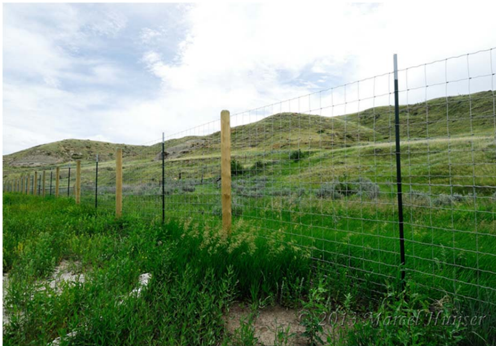
Figure 30: A 2.4 m high wildlife fence, designed to be a barrier to ungulates such as deer ( Odocoileus spp.) and pronghorn ( Antilocapra americana ), Hwy 2, near Havre, Montana, USA (© Marcel Huijser).
