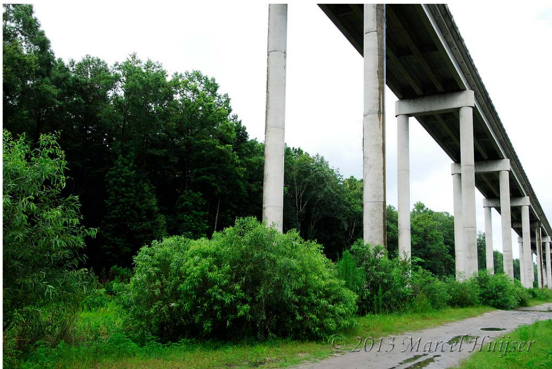
Figure 24: Elevated roadway, central Florida, USA (© Marcel Huijser).
