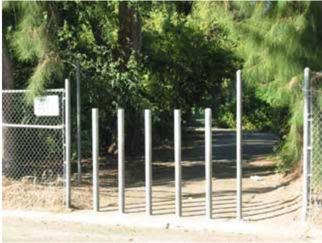
Figure 33: Aluminum fence posts (Source: Ed Cox).
