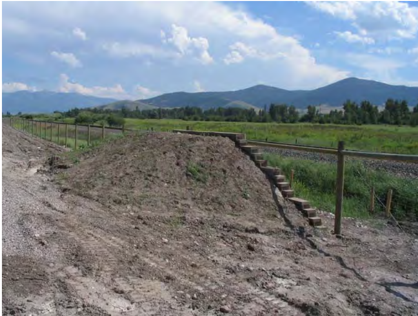
Figure 33. A jump-out along a 2.4 m (8 ft) high fence along US 93 in Montana, USA (© Marcel Huijser).
