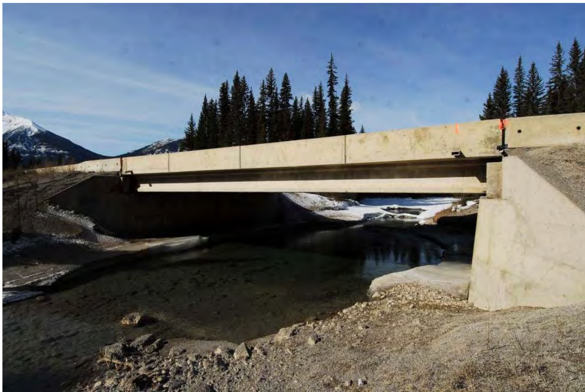
Figure 63. The bridge across the Kootenay River at Kootenay Crossing (© Marcel Huijser).
