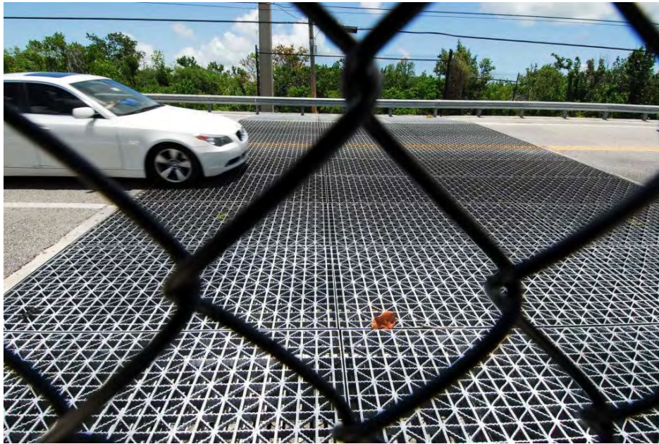
Figure 32. Wildlife guard at a fence end on the 2-lane US Hwy 1 on Big Pine Key, Florida, USA (© Marcel Huijser).
