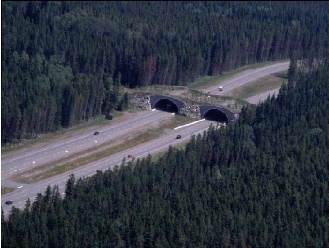
Figure 44. Red Earth overpass on the Trans-Canada Highway (© Tony Clevenger, WTI).
