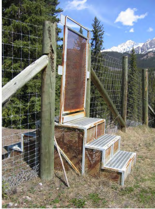
Figure 40: Swing gate in fence (spring loaded) allowing access for people, also when there is snow on the ground, along the Trans-Canada Highway in Banff National Park, Alberta, Canada (© Adam Ford, TCH research project / WTI-MSU).
