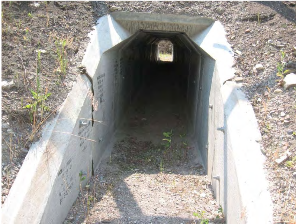
Figure 48. A medium mammal box culvert (1.2 m wide, 1.8 m high) along the 2-lane US Highway 93 on the Flathead Reservation in Montana, USA (south of Ravalli) (© Marcel Huijser).
