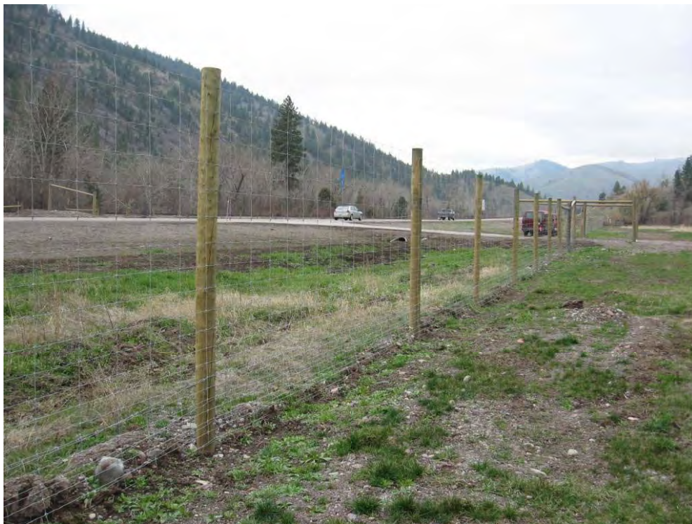
Figure 28. A 2.4 m high wildlife fence along the 2-lane US Highway 93 on the Flathead Reservation in Montana, USA (© Marcel Huijser, WTI-MSU).
