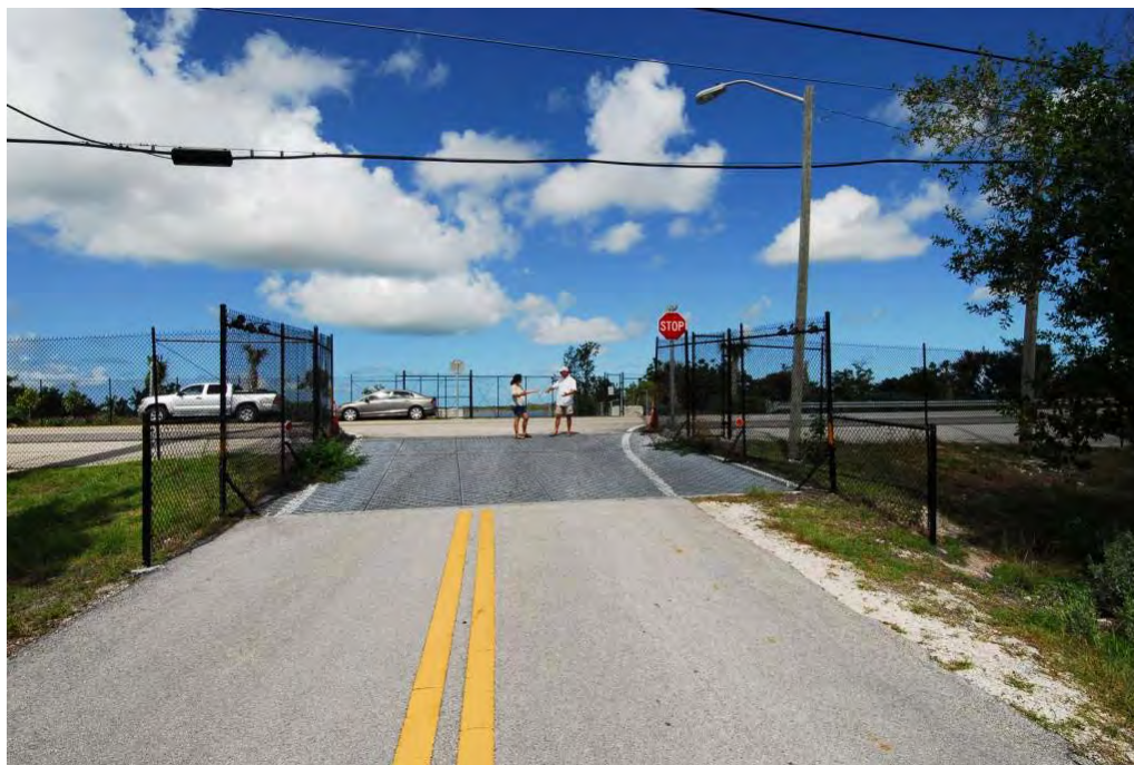
Figure 37. A wildlife guard at an access road of the 2-lane US Highway 1 on Big Pine Key, Florida, USA (© Marcel Huijser)
