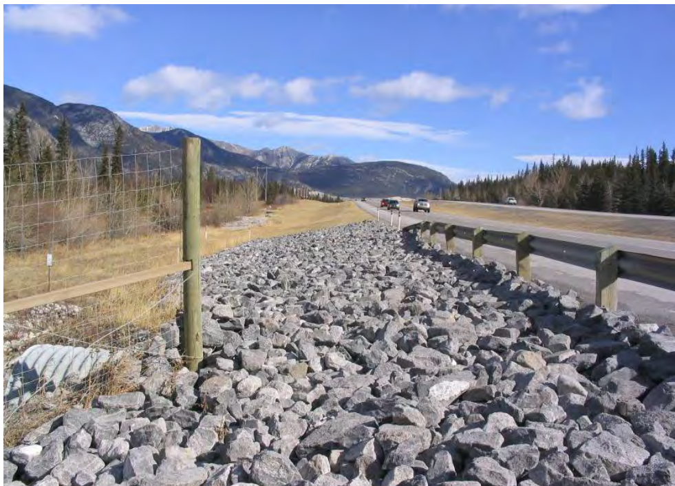
Figure 31. The Boulder Field at the Fence End at Dead Man's Flats Along the Trans Canada Highway East of Canmore, Alberta, Canada (© Bruce Leeson).
