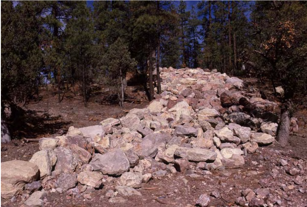
Figure 29. Large boulders placed in the right-of-way as a barrier to elk and deer along State Route 260 in Arizona, USA (© Marcel Huijser).
