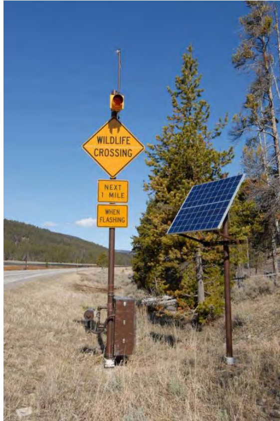
Figure 52. An animal detection system (microwave radio signal break-the-beam system manufactured by Sensor Technologies & Systems, Scottsdale, AZ) installed along a 1 mile (1,609 m) section of US Hwy 191 between Big Sky and West Yellowstone in Yellowstone National Park (© Marcel Huijser, WTI-MSU).
