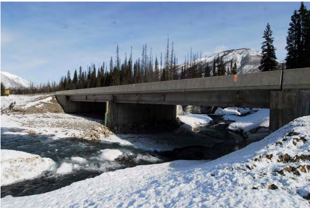
Figure 65. The bridge across the Vermilion River at Vermilion Crossing (© Marcel Huijser).
