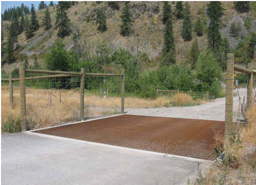
Figure 36. A wildlife guard at an access road of the 2-lane US Highway 93 on the Flathead Reservation in Montana, USA (© Marcel Huijser)
