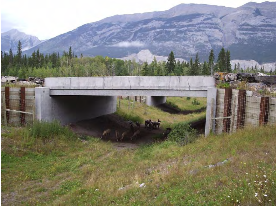
Figure 59. Bighorn sheep using an underpass, and licking minerals, along the Trans-Canada Highway near Canmore, Alberta, Canada. (© Tony Clevenger).
