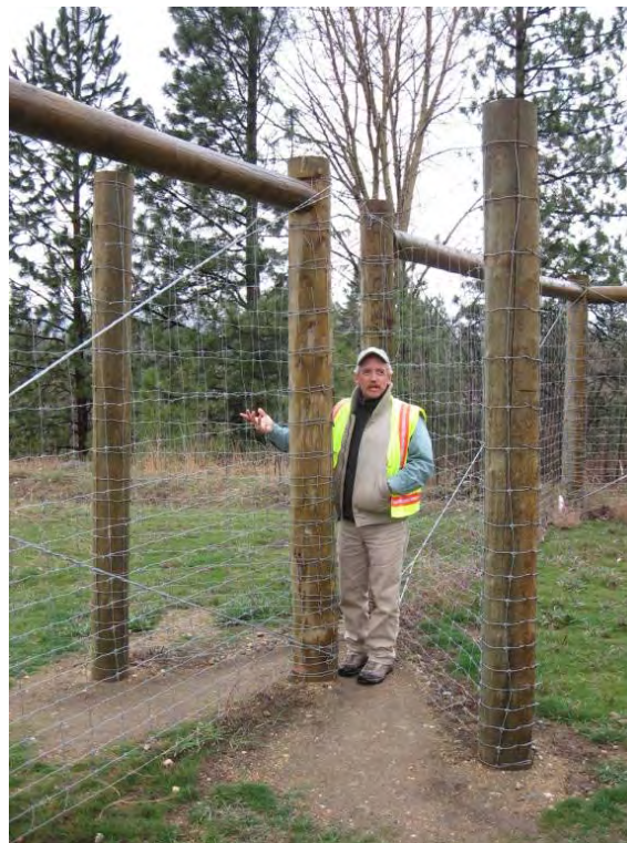
Figure 41: Access point for people along US93, south of Missoula, Montana, USA (© Marcel Huijser). This type of gate may be a barrier for ungulates.
