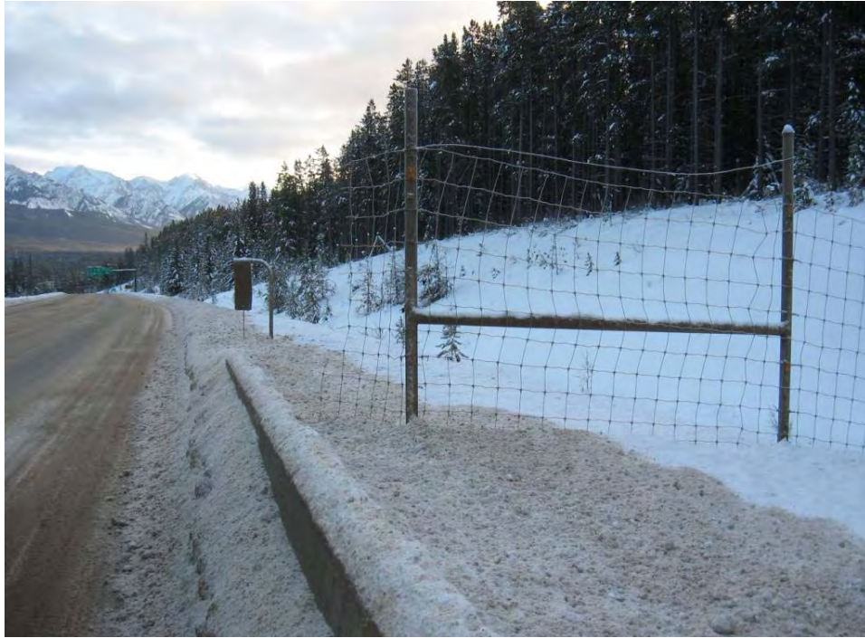
Figure 30. Fence end brought close to the road with a concrete barrier for safety along Hwy 93S in Banff National Park, just west of Castle Jct (© Marcel Huijser, WTI-MSU).
