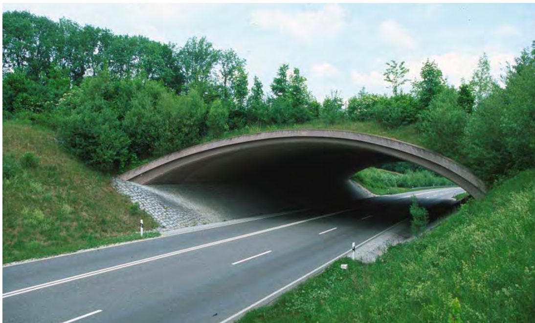
Figure 45. Wildlife overpass (“Schwarzgraben”) across a 2-lane road (B31) in southern Germany (© Edgar van der Grift).
