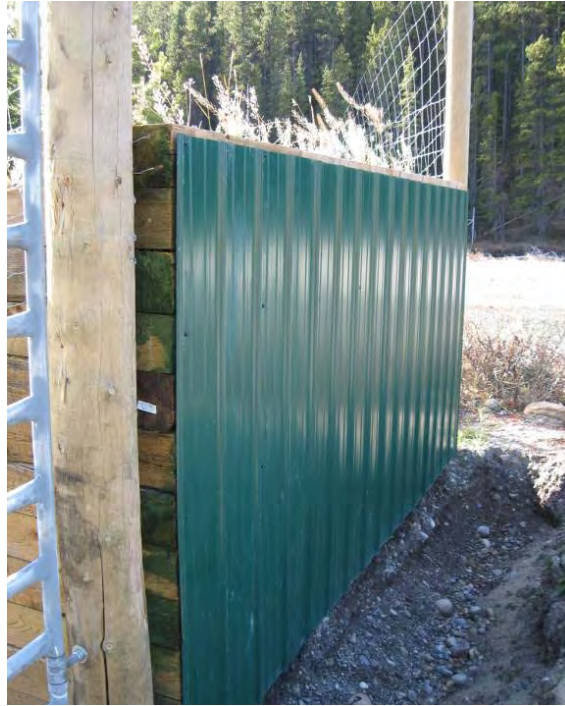
Figure 35. A jump-out along a 2.4 m (8 ft) high fence with smooth metal to prevent bears from climbing the jump-out the wrong way. Along the Trans Canada Highway, Lake Louise area, Banff National Park, Canada (© Marcel Huijser, WTI-MSU).
