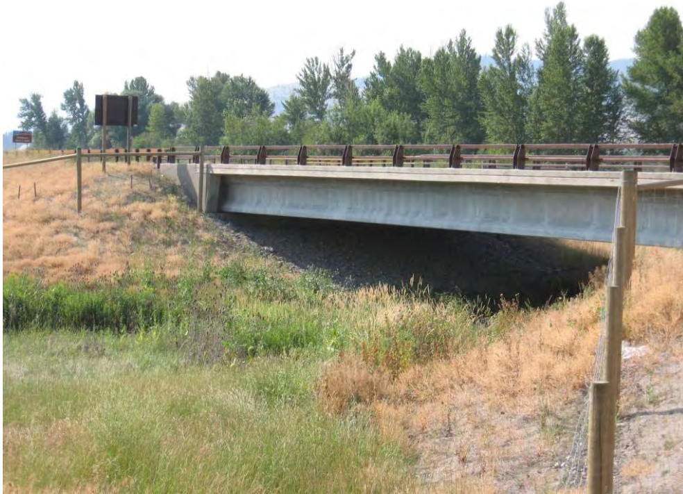
Figure 46. An open span bridge along the 2-lane US Highway 93 on the Flathead Reservation in Montana, USA (across Spring Creek, south of Ravalli) (© Marcel Huijser).
