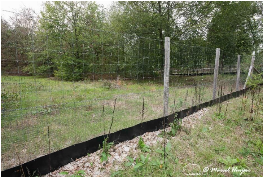
Figure 7: Wildlife fence for large mammals (e.g., roe deer ( Capreolus capreolus )) (tall wire mesh), medium mammals (smaller mesh size towards bottom) (e.g., Eurasian badger ( Meles meles )), and small animal species (smooth black plastic sheets that extend into the soil), including amphibians, reptiles, and small mammal species. This fence keeps wildlife from accessing a railroad (three tracks) and guides them toward the wildlife overpass "Op Hees" across the railroad tracks between Utrecht and Soest/Amersfoort, Soest, The Netherlands.
