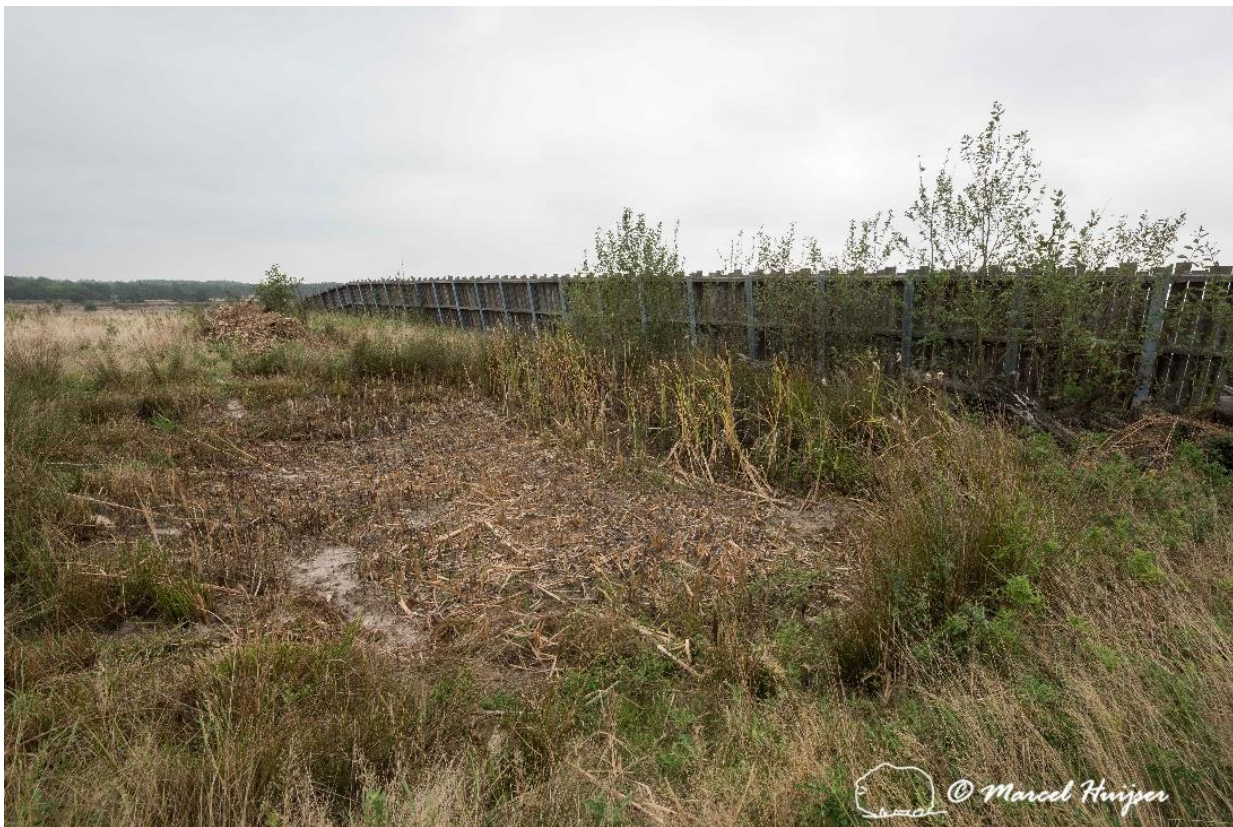
Figure 3: Pool (during dry time of the year) on top of wildlife overpass “Groote Heide” across A2 motorway, near Leende, The Netherlands. This pool is a stepping stone for the following target species for this overpass: moor frog ( Rana arvalis ), great crested newt ( Triturus cristatus ).
