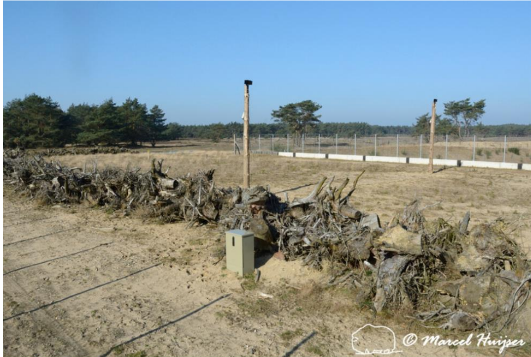
Figure 1: The top of a designated wildlife overpass for species associated with dry forests, heathlands, and inland sand dunes. Note the wildlife cameras, the sparse vegetation characteristic of this type of habitat, and root wads on top of wildlife overpass Oud Reemst, south of Otterlo, The Netherlands.
