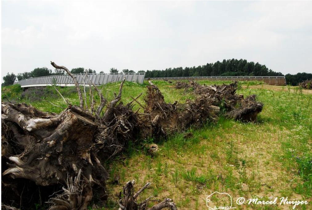
Figure 4: A row of root wads on an approach of a wildlife overpass guides small animal species dependent on cover across the structure, Ecoduct “Waterloo” across A73 motorway near Roermond, The Netherlands.
