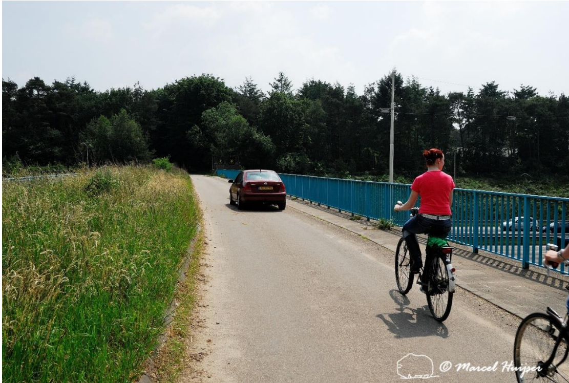
Figure 2: This overpass was originally a two-lane bridge for pedestrians, cyclists, and cars across a motorway. Much later, about half the width was made into a “nature strip” with some soil, root wads, grasses, herbs and shrubs. This is an example of an overpass, originally built for other purposes than wildlife, that was modified for wildlife later. The Netherlands.
