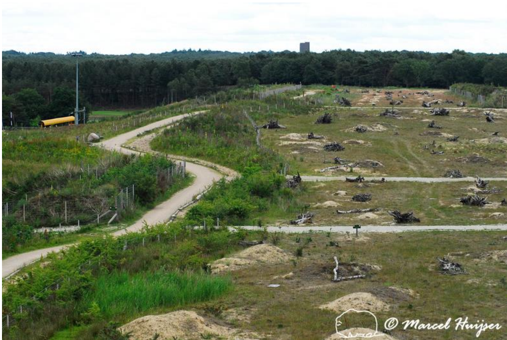
Figure 5: Open habitat (sandy spots, grass herb vegetation) and cover (stacks of root wads) on wildlife overpass “Zanderij (Crailoo)”, near Hilversum, The Netherlands. The structure connects forests and heath lands, is 800 m long, 50 m wide and crosses a 2-lane road, a 2-track railroad, a railroad yard, and a golf course and field hockey complex. Among the target species currently present in the area, are two lizard species, 1 snake species, 2 frog species, 2 toad species, 1 newt species, and a range of small-medium sized mammal species. Note that there is also a trail for non-motorized traffic on this overpass. More information on the effectiveness of this overpass in van der Grift et al. (2009).
