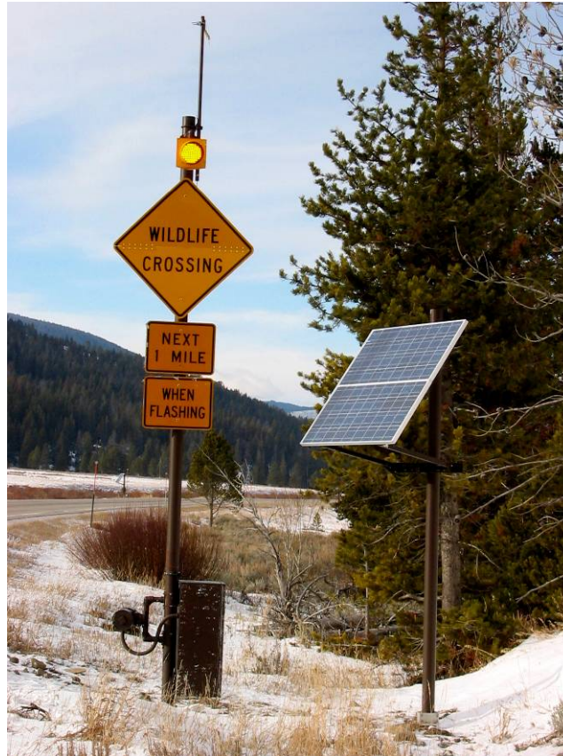
Figure 14. An animal detection system on US Highway 191 in Yellowstone National Park, Montana. Photo by Marcel Huijser, WTI.
