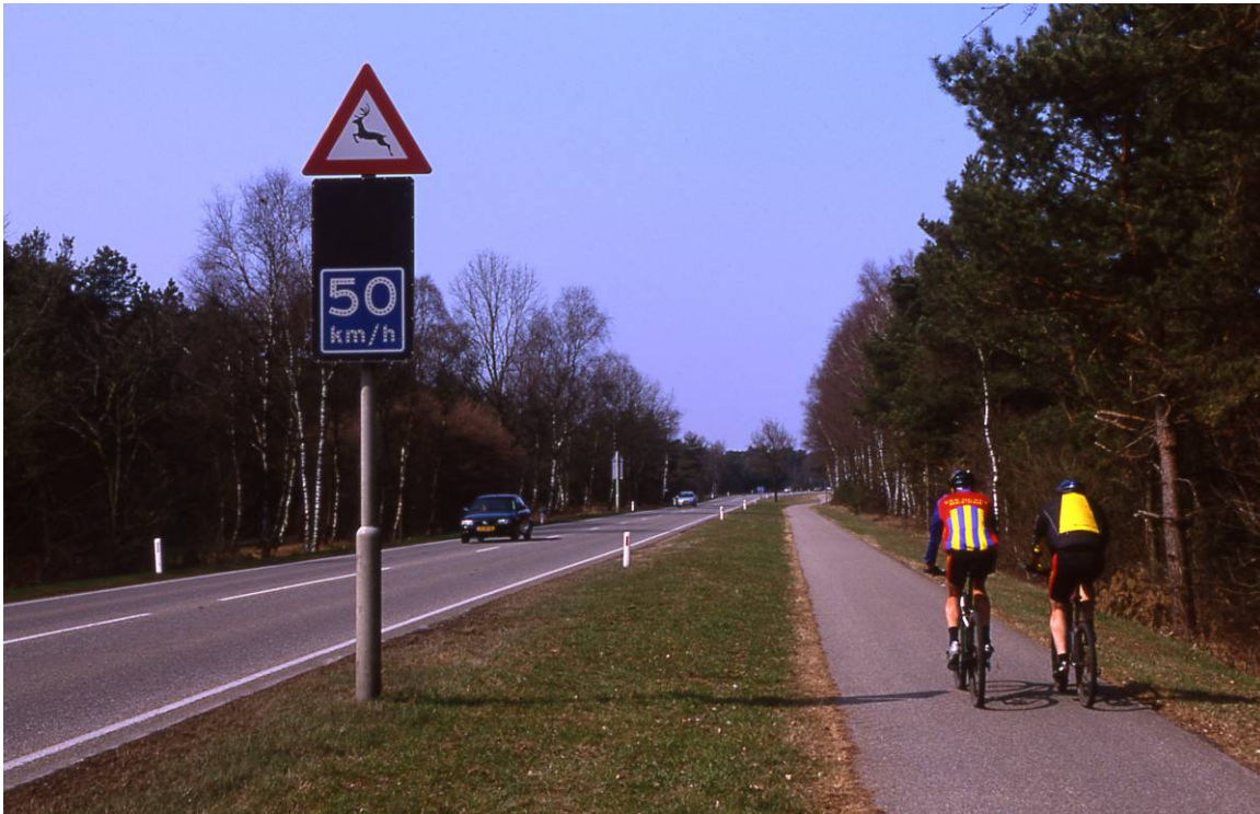
Figure 4. Advisory speed limits accompany a deer warning sign near 't Harde, The Netherlands. Note: The LED part of the warning sign is linked to an animal detection system, but the advisory speed limit reduction sign is always visible in daylight, regardless of the presence and detection of large animals. Photo: Marcel Huijser.
