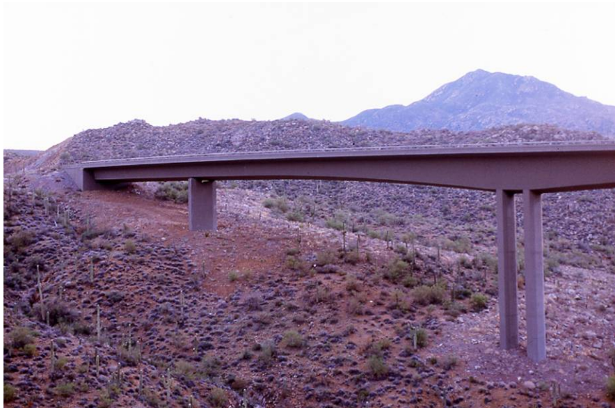
Figure 22. A long bridge on State Route 260 in Arizona. Photo by Marcel Huijser.
