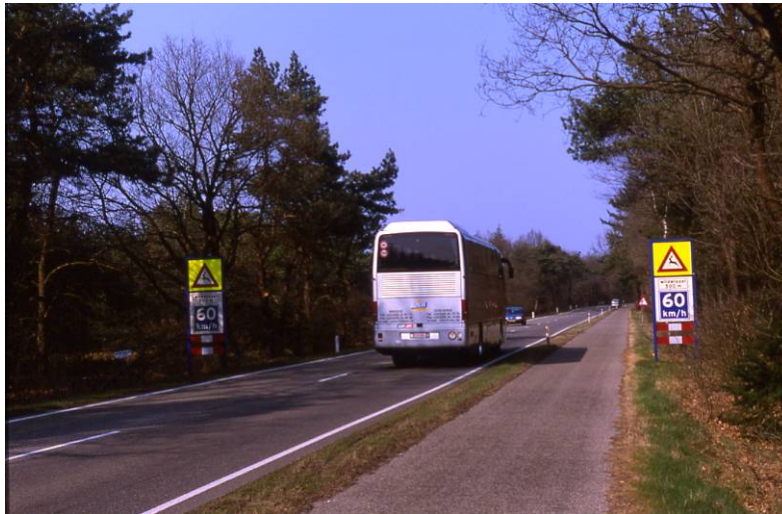
Figure 24. Advisory speed limit reduction at a fence gap where large animals (red deer, wild boar, roe deer) may cross at grade in The Netherlands. Photo by Marcel Huijser.
