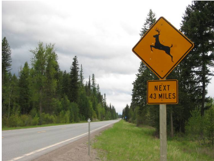
Figure 7. Standard deer warning sign on MT 83 in Montana accompanied by the length of the road section that the warning sign applies to. Photo by Marcel Huijser, WTI.
