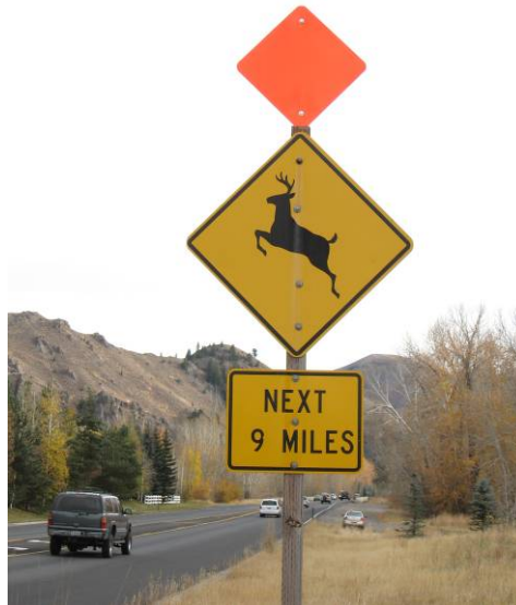
Figure 8. Enhanced standard deer warning sign on State Highway 75 in Idaho. Photo by Marcel Huijser, WTI.
