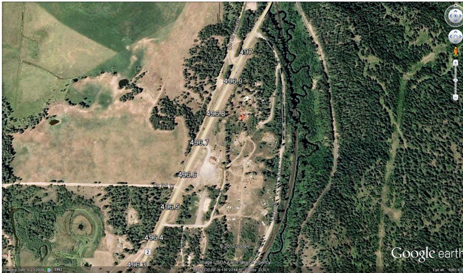
Figure 34. The Hwy 95 494.8-497.1 hotspot showing the 0.1 mi markers on a satellite image background.
