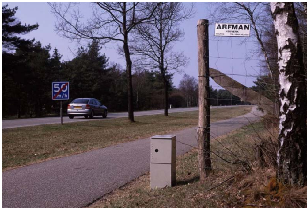
Figure 29. An animal detection system (infrared break-the-beam system manufactured by Calonder Energy, Switzerland) at a gap in a wildlife fence near 't Harde, The Netherlands (© Marcel Huijser).
