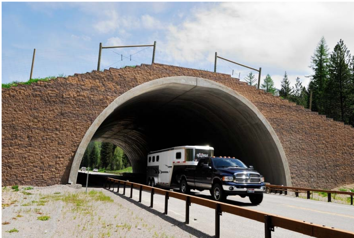
Figure 23. Wildlife overpass across a 2-lane road (US Hwy 93) on the Flathead Indian Reservation, Montana, USA (© Marcel Huijser).
