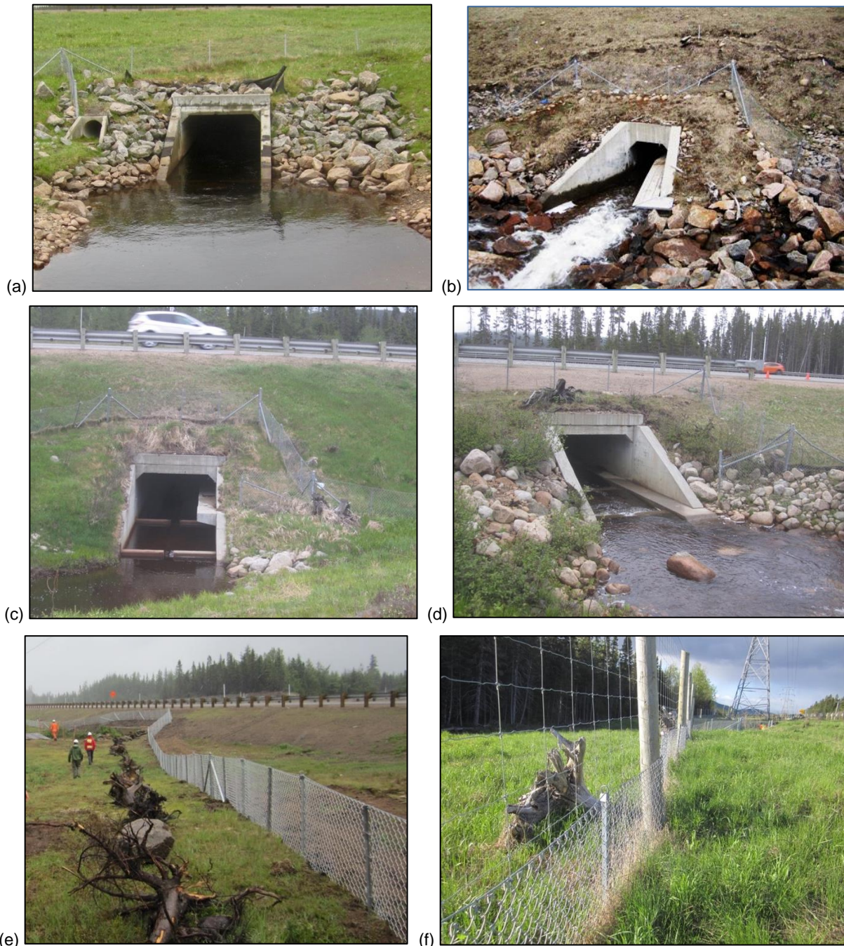
Figure 3: The four types of wildlife underpasses designed for small and medium-sized mammals and the two types of fences along Highway 175: (a) pipe culvert or round concrete culvert (on the left next to the water culvert; n = 6 ), (b) box culvert with a wooden ledge ( n = 4 ), (c) box culvert with a concrete ledge ( n = 7 ), (d) box culvert with a concrete walkway ( n = 1 ), (e) fence for medium-sized mammals, and (f) combined fencing for large mammals (upper half) and medium-sized mammals (lower half). Photo Credit: Concordia University Montreal, J. Jaeger.
