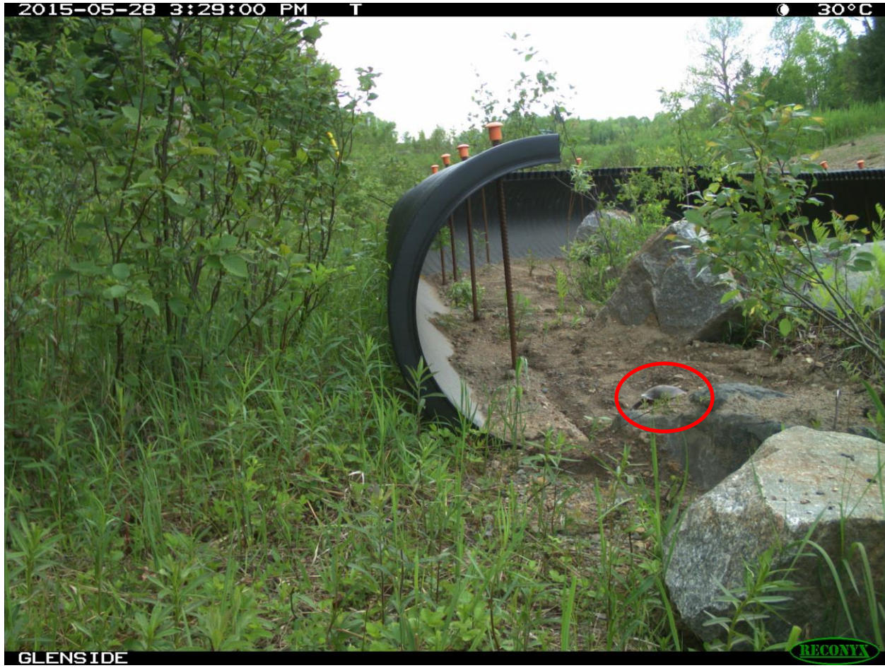
Figure 7: Curved back barrier ends that redirected at least 23% of the turtles back towards the drainage culvert; turtle shown in red circle. Photo Credit: Paul Heaven.
