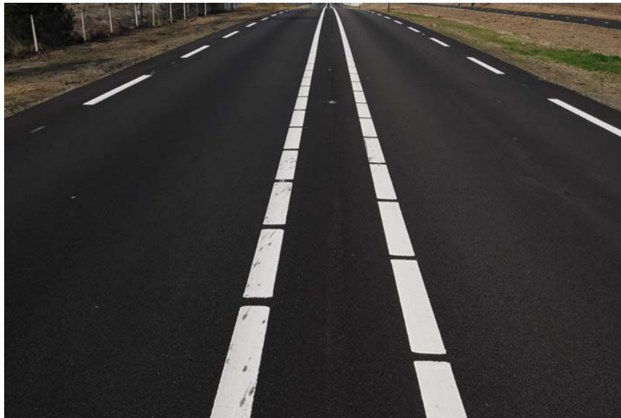
Figure 4.1: Wider and double striping along the edges and center of a road in The Netherlands resulting in narrower lanes, and potentially lower vehicle speeds, without reducing the actual width of the road (© Marcel Huijser).
